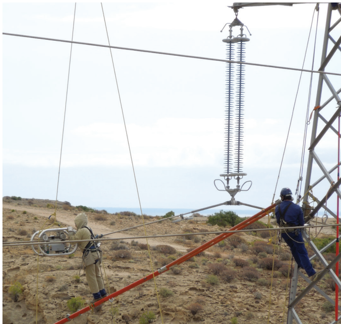
Installation from Ropes/Ladders
