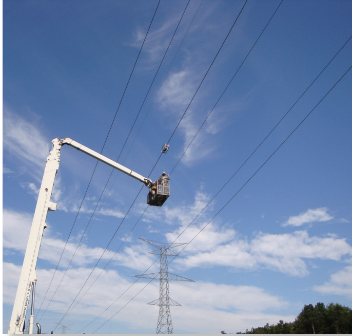
Installation from Bucket Trucks
