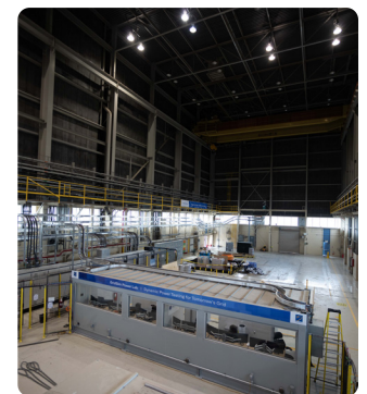
GridSim Power Lab
