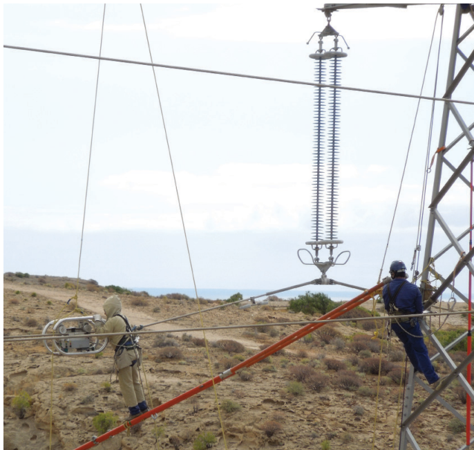
Installation from Ropes/Ladders
