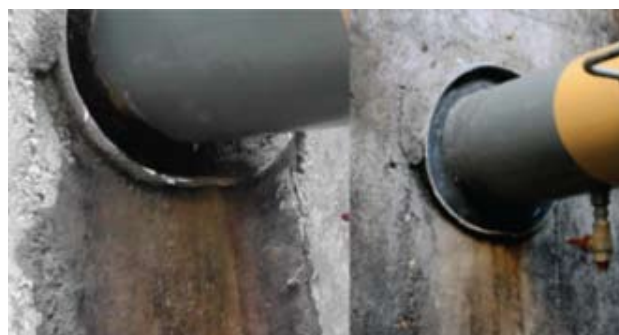
Pipe penetration before and after fitting of an annular seal.
