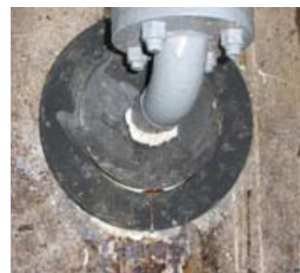
Preformed water blocking gasket after fitting.
