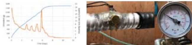
Figure 2. (Left) Leak / time chart for ANAGEN™ in open air showing complete leak cessation. (Right) Image following test completion showing build-up of cured material on leak site. Cable pressure constant at 30 PSI.
