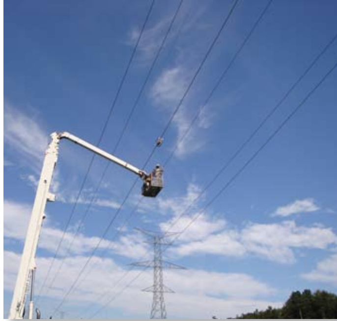
Installation from Bucket Trucks
