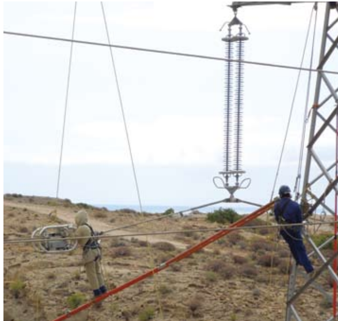
Installation from Ropes/Ladders
