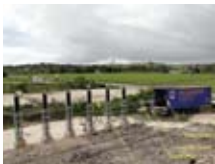
Kinectrics' mobile Resonant Test System (RTS)
