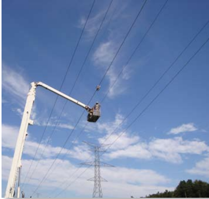
Installation from Bucket Trucks
