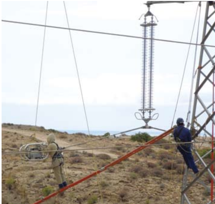
Installation from Ropes/Ladders
